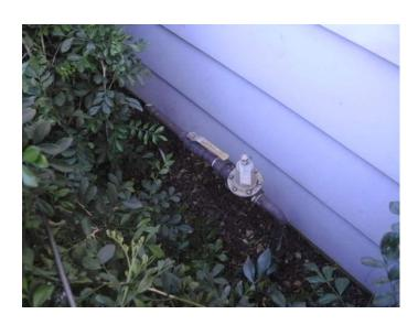
**Comments:** A pressure regulator located at the shutoff valve at the left side of the home controls the pressure to 90 p.s.i.
