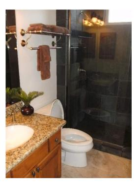
■ Recommend caulking at the bottom of the shower glass panel. Recommend ensuring the integrity of the caulking and grout at all water related areas and this should be considered part of a regular maintenance program.
