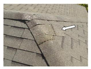
• An exposed nail was noted at the back of the roof. Recommend sealing the exposed nail with roofing cement to prevent moisture infiltration.
