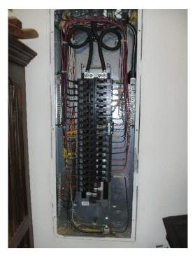
Comments: AFCI (Arc Fault Circuit Interrupter) protected outlets were noted at the outlets in bedroom #2 and #3. AFCI's are a relatively new safety feature for residential construction that protects the bedrooms of a home from defective wiring or appliances by shutting off the circuit when a defect is noted. The overall condition of the sub-panel was noted to be good, although:
