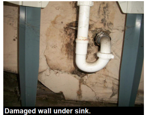
Damaged wall under sink.
