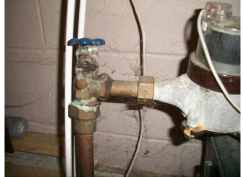
Corroded shut off valve.
