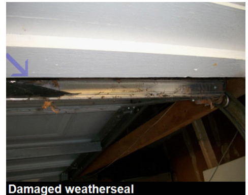
Damaged weatherseal
