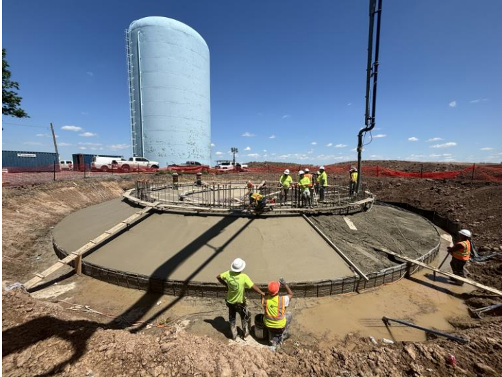
Brickyard Road Tank base being poured
