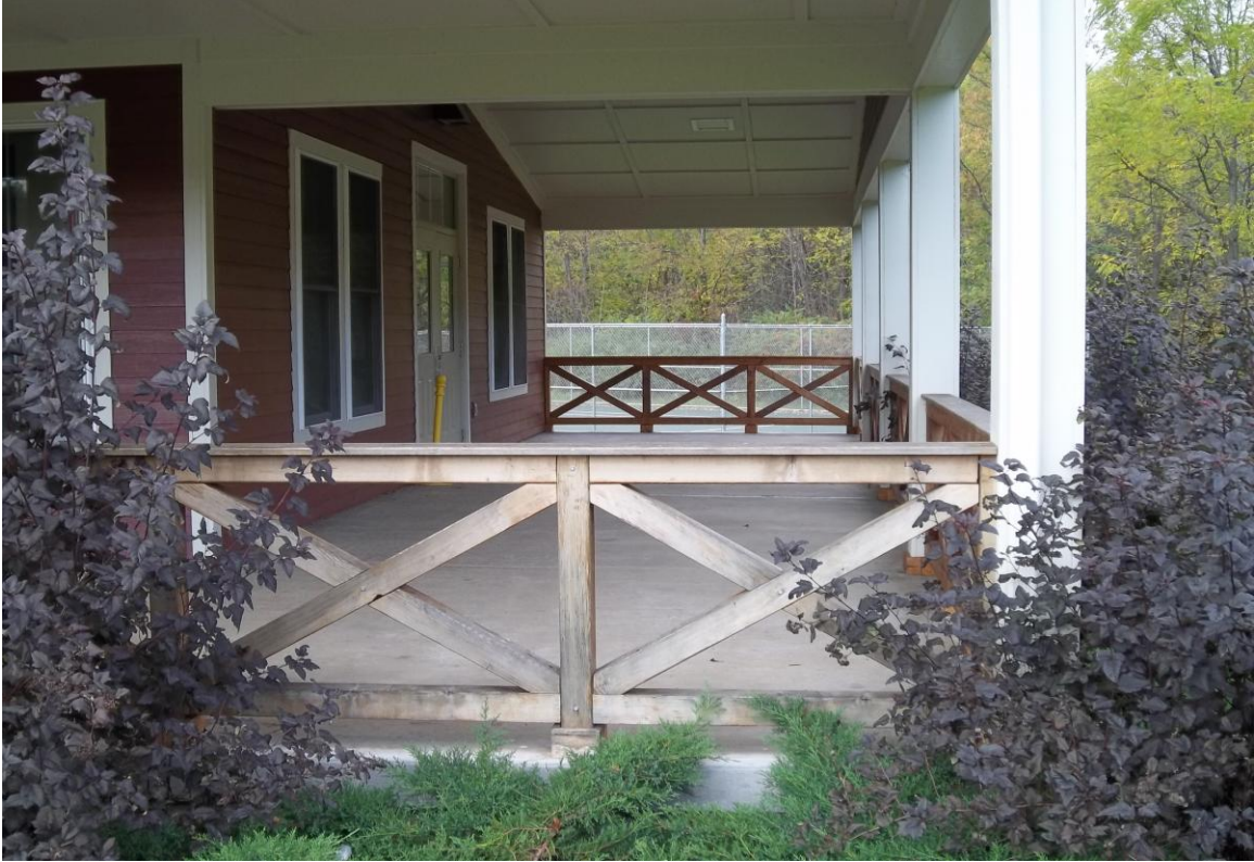
Back Porch Area of Mertensia Lodge
