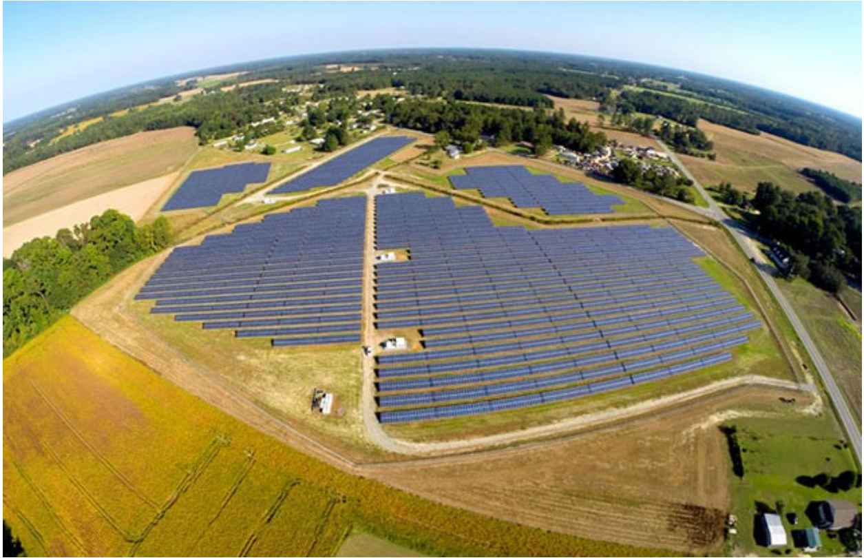
6.5MW system – S-Power, Fairmont, North Carolina
