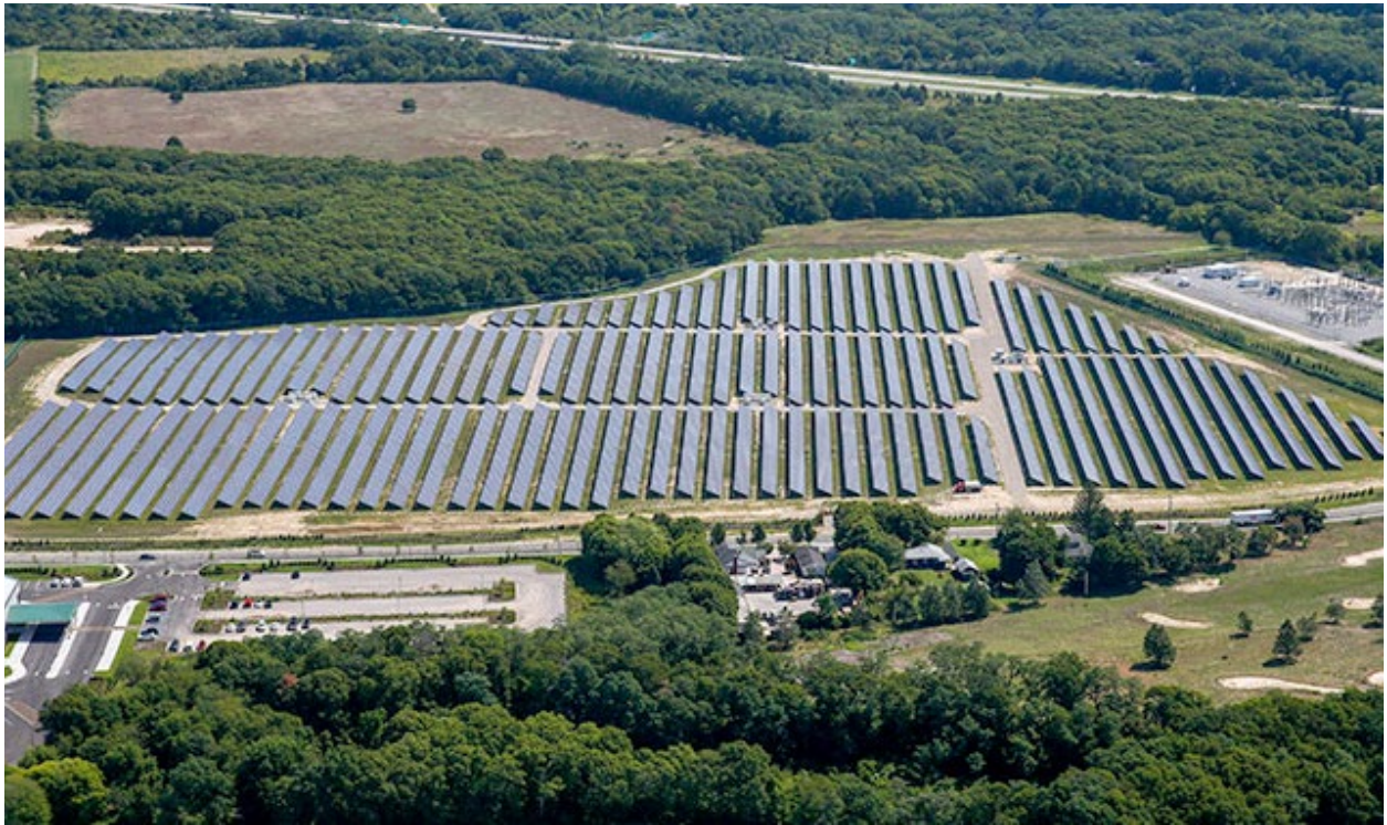
9.2MW system – S-Power, Calverton, New York
