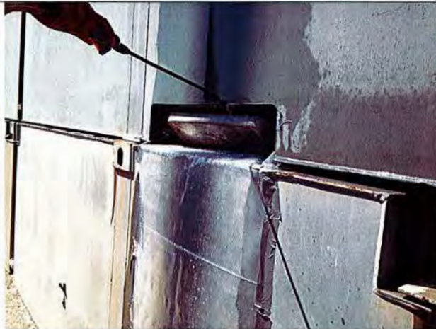
Causeway, portion with zinc anode; Little Creek
