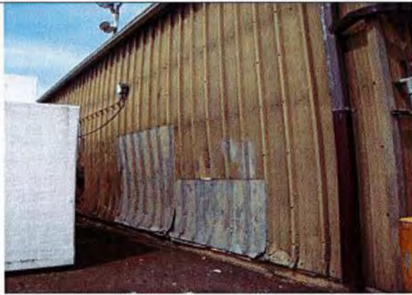
Galvanize siding, painted, chipped; NBK Bangor
