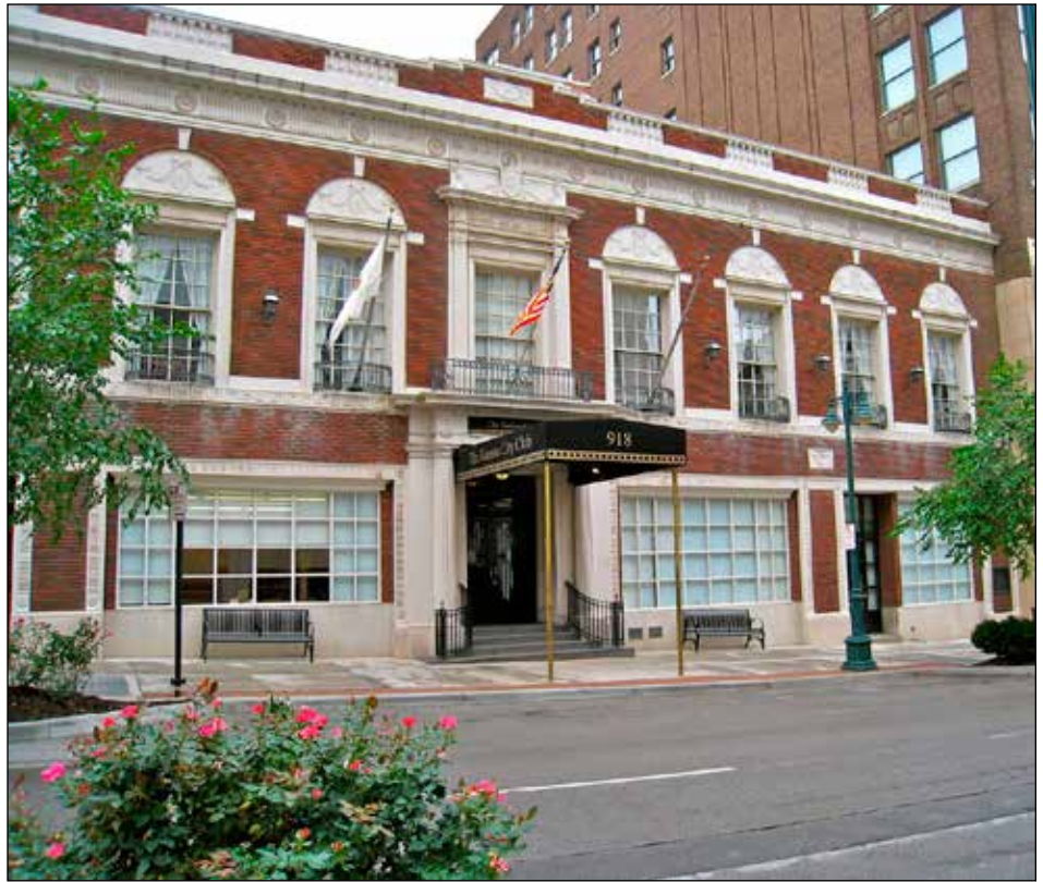
Kansas City Club is located at 918 Baltimore Avenue in downtown Kansas City.
