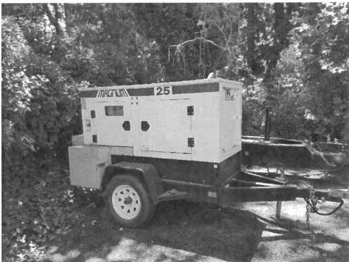
Magnum 25A Trailer Mounted Generator
