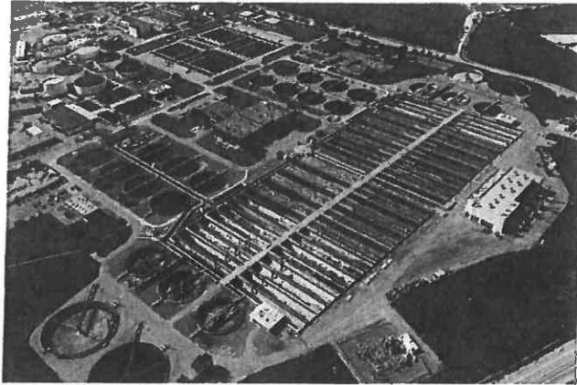
San José-Santa Clara Regional Wastewater Facility
