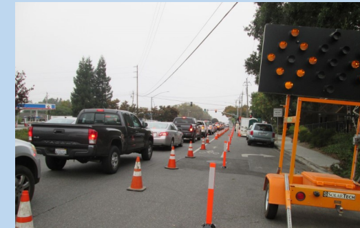
Traffic control in place during construction
