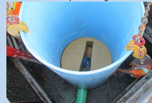
Three new plastic wetwells installed
