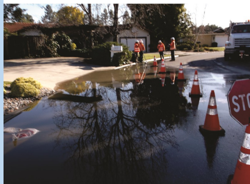
Sanitary sewer spills due to pump failure
