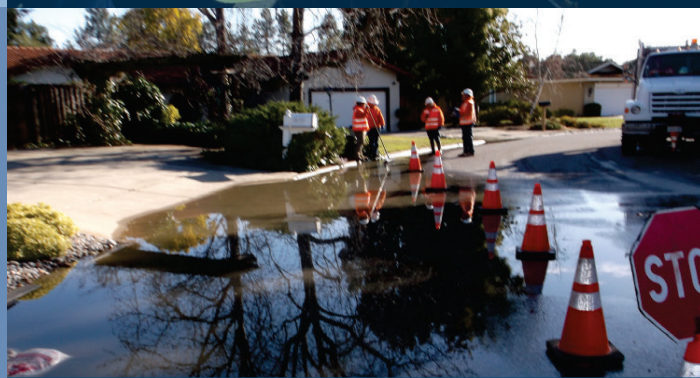
Sanitary sewer spills due to pump failure
