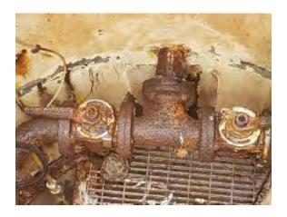
Forum 2 Pump Station requires replacement of the quick connector adaptor hook up hose to exercise force main and gate valve.
