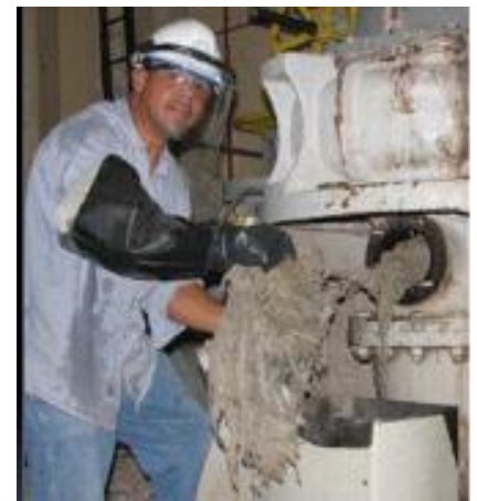
Utility workers are also placed at risk of physical injury and illness from removing sewage-soaked wipes from equipment.
