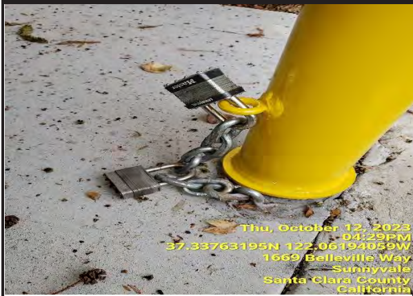
Eye hooks installed to hold bollards in place
