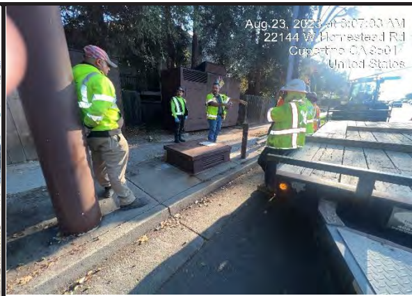
Generator Removal Safety Meeting
