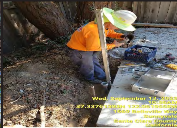
Super Strut Being Anchored and Bolted into the Slab
