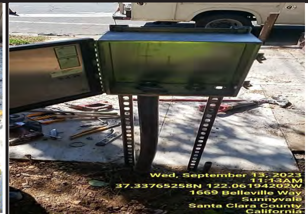
J Box is installed, Ready to be Wired Up
