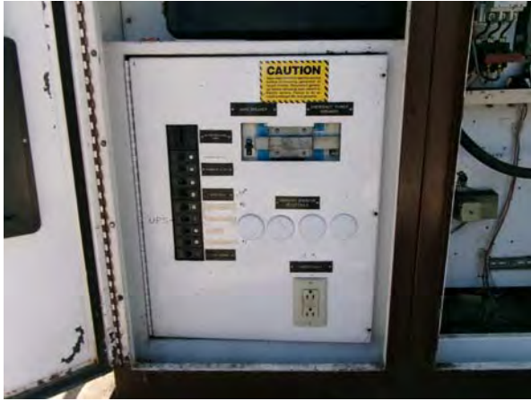
Replace Generator Breaker
