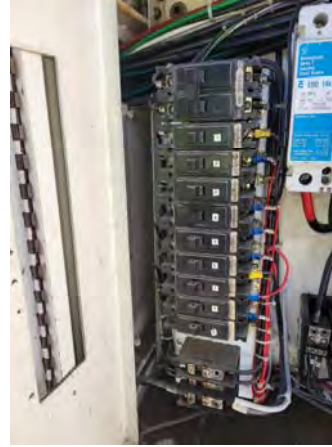
Replace Circuit 3 with Tandem Breaker
