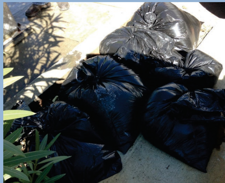
Five bags of wipes and debris from pump station cleaning
