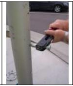
Using the expanding rivet nut tool, install the rivet nuts into the pole. See rivet nut manufacturer for proper sized hole as the rivet nuts must fit tightly in the holes in order to hold properly.
