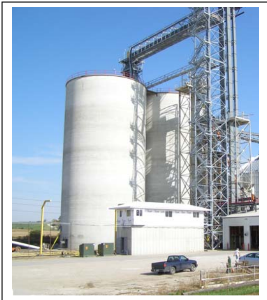
Slip form concrete grain silos
