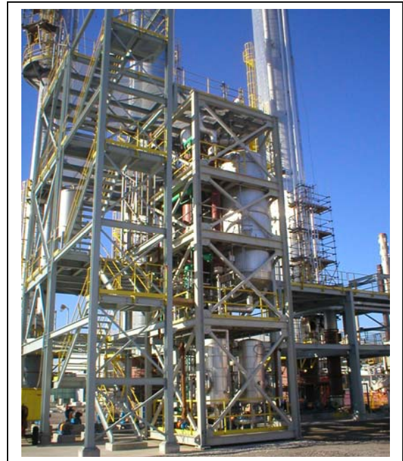
Erected on site with mating stair tower (on left)
