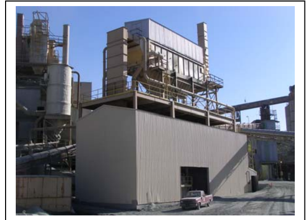
Overall view of dryer building and bag house mounted above the structure.
