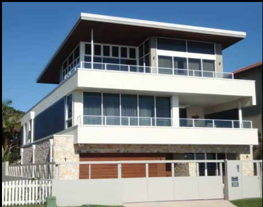
▲ Billinga Beach House is a 3 level house built to take advantage of its surroundings.
