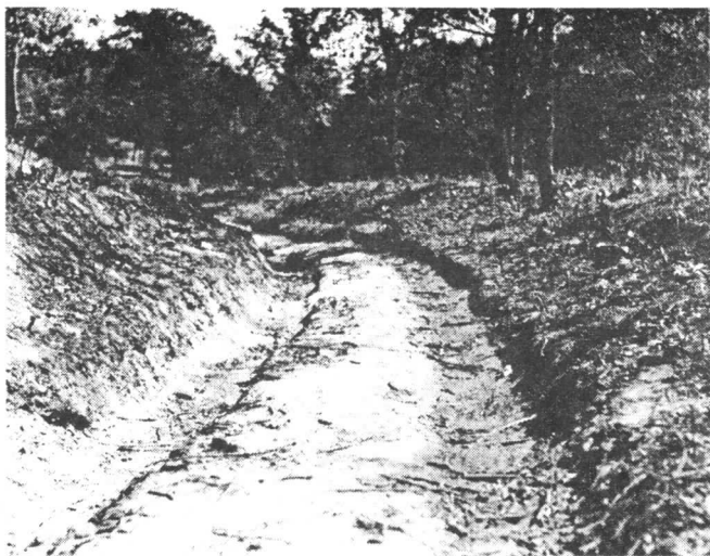
Road from the Bluff to the Independence / Wayne City Landing - photo from the C. Ed. Miller collection.
