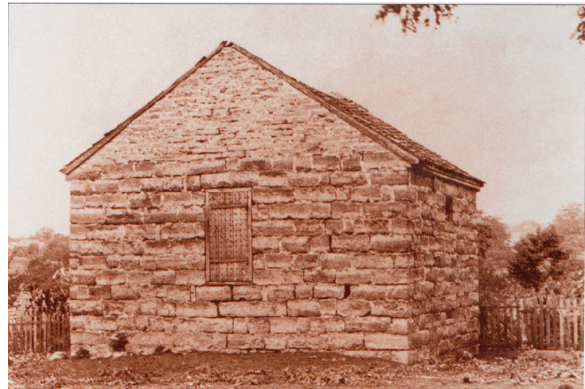
The abandoned Liberty Jail photo by Hicks
