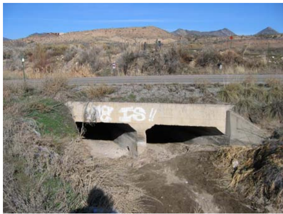
Photo 2 – Double Cell 6' x 4' Concrete Box Culvert – Lower Cactus Valley Ditch
