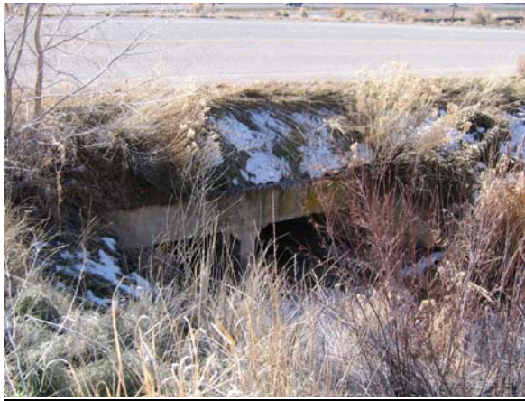
Photo 4 – Double Cell 6' x 4' CBC at the outlet west of Davis Point.
