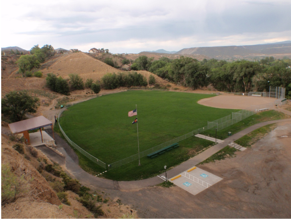
Stoney Ridge Ball Field/Pavilion, including parking areas, loading/unloading zone
