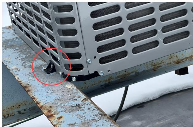
Figure 6. Example rigid connections to rooftop CU and dunnage
