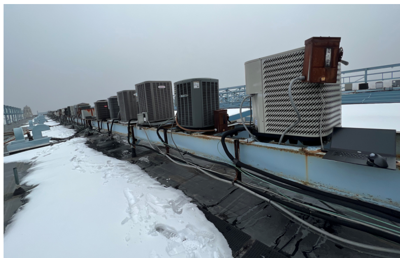
Figure 3. Northern row of rooftop CUs
