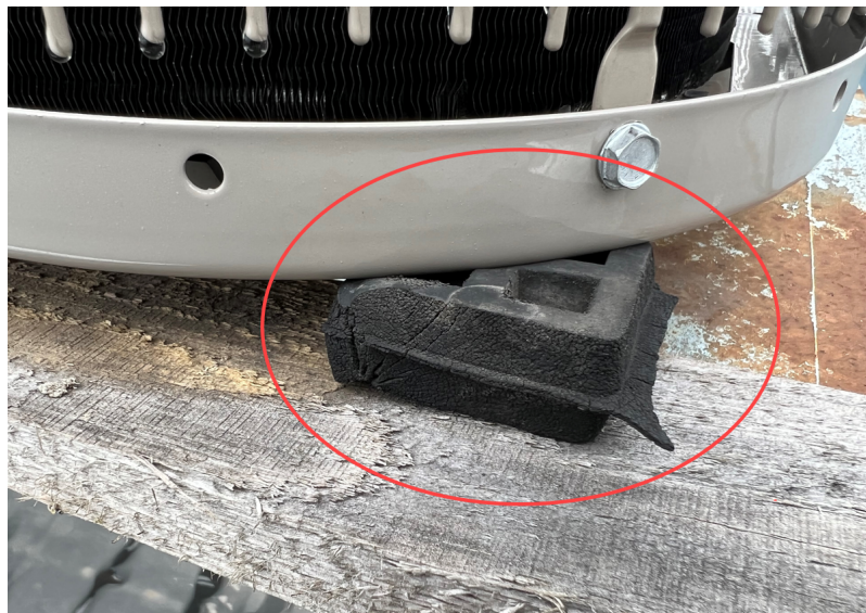
Figure 2. Example of vibration isolator installation beneath CU
