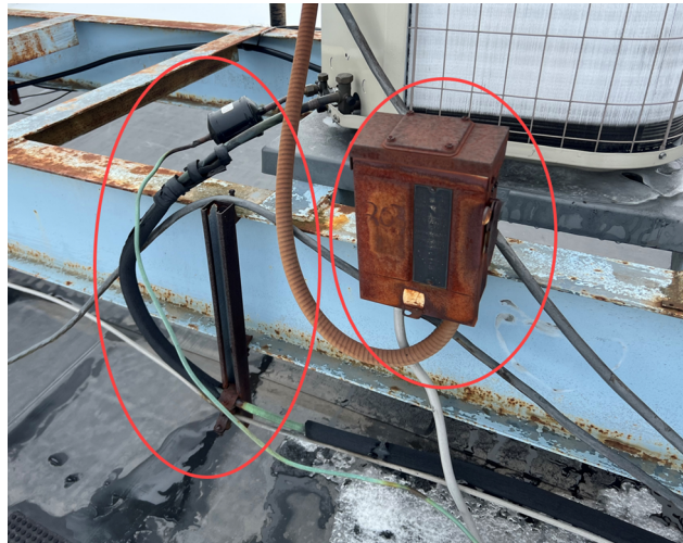
Figure 5. Example rigid connections to rooftop CU and dunnage
