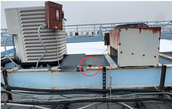
Figure 9. Node 3874 attached to CU dunnage
