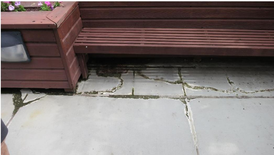
*Photo 4. Deterioration at lower atrium topping slab*
