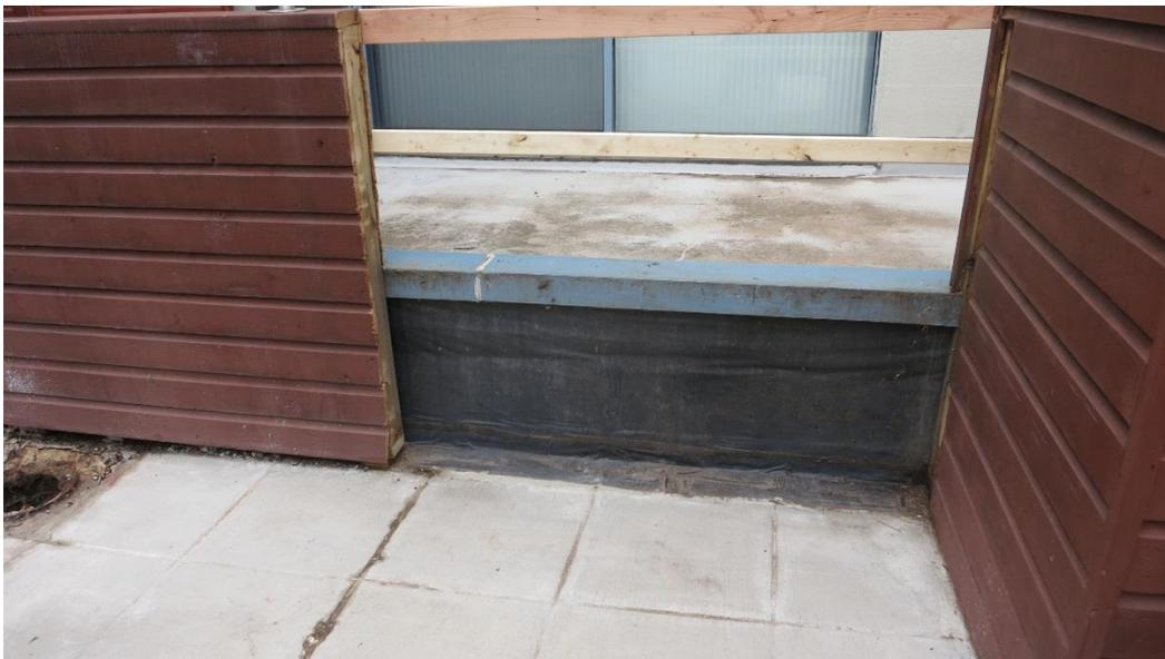
*Photo 8. Probe 1- cut open planter wall at Unit 235*
