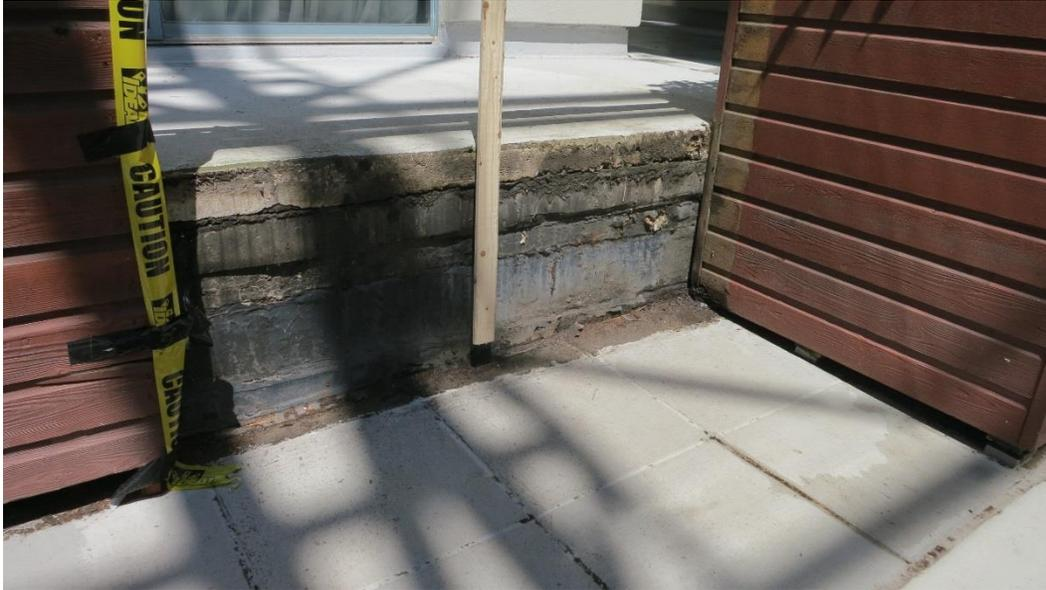
*Photo 23. Probe 14 - Patio wall removal at Unit 215*
