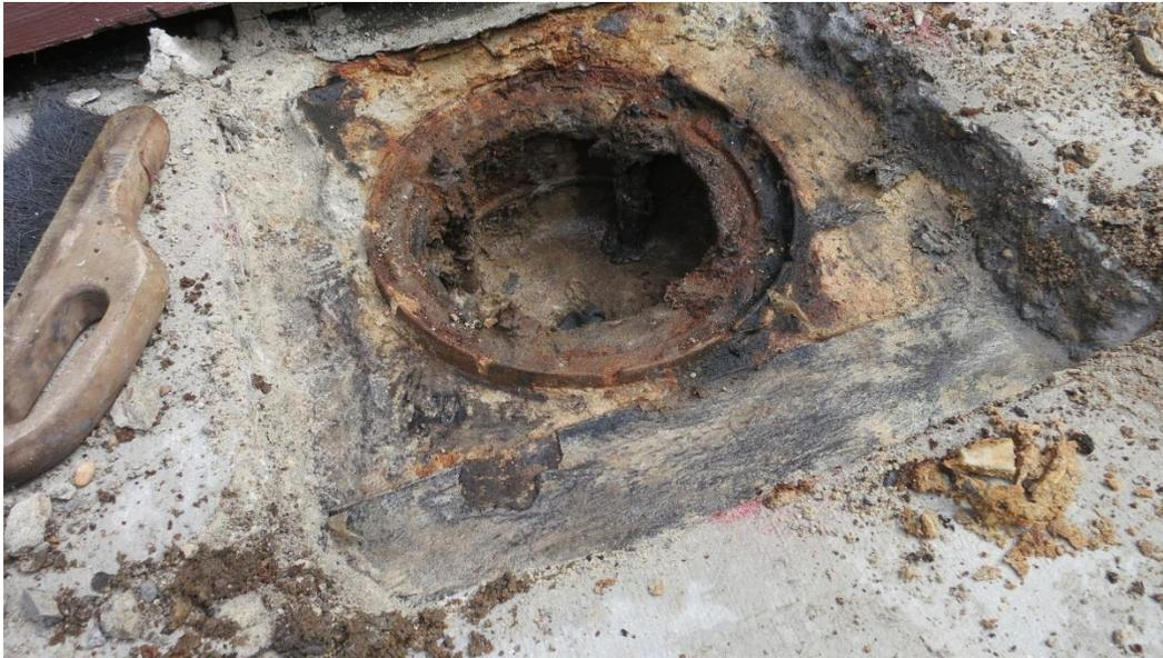
*Photo 9. Probe 1a - Cut open floor drain at Atrium lower level slab.*
