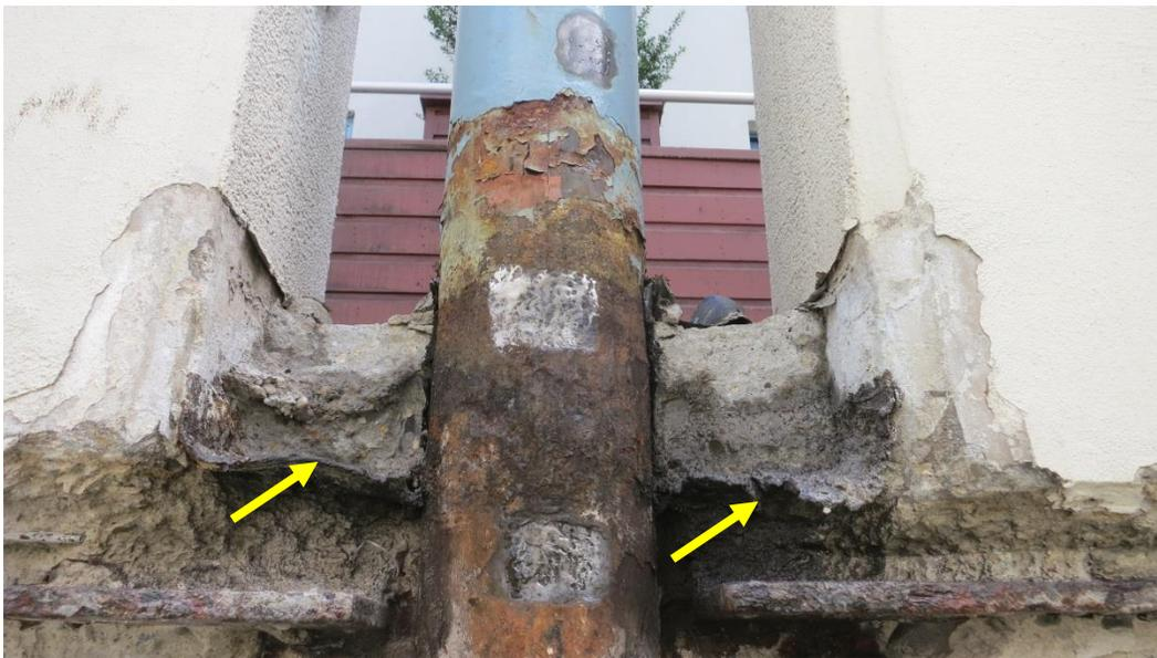
*Photo 24. Membrane ends inside lightwell wall with no termination.*
