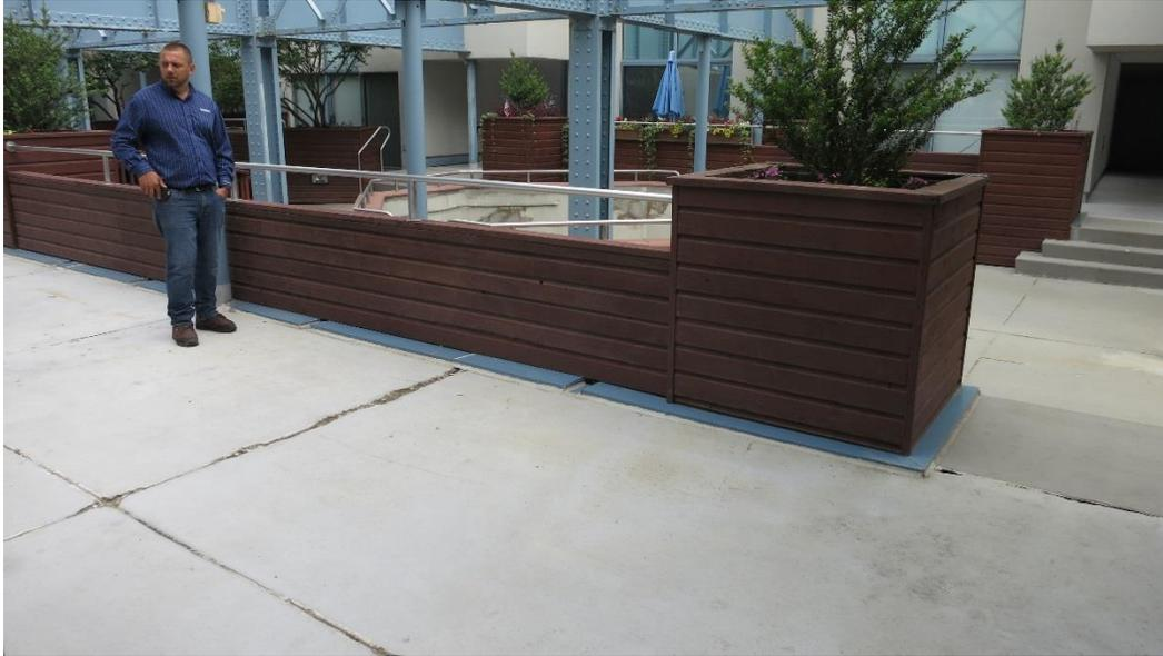
*Photo 5. Minor deterioration at joints in upper atrium slab*
