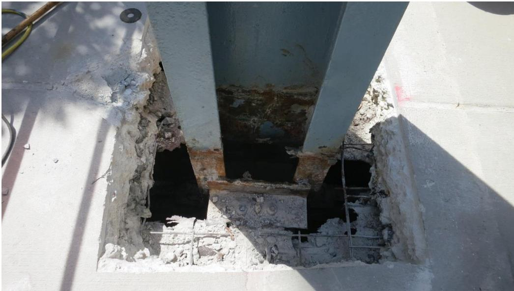
*Photo 14. Probe 5 - Full depth concrete removal at column*
