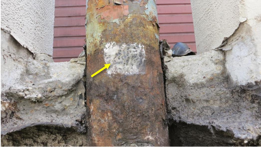
*Photo 25. Portion of hanger ground clean for thickness measurement.*
