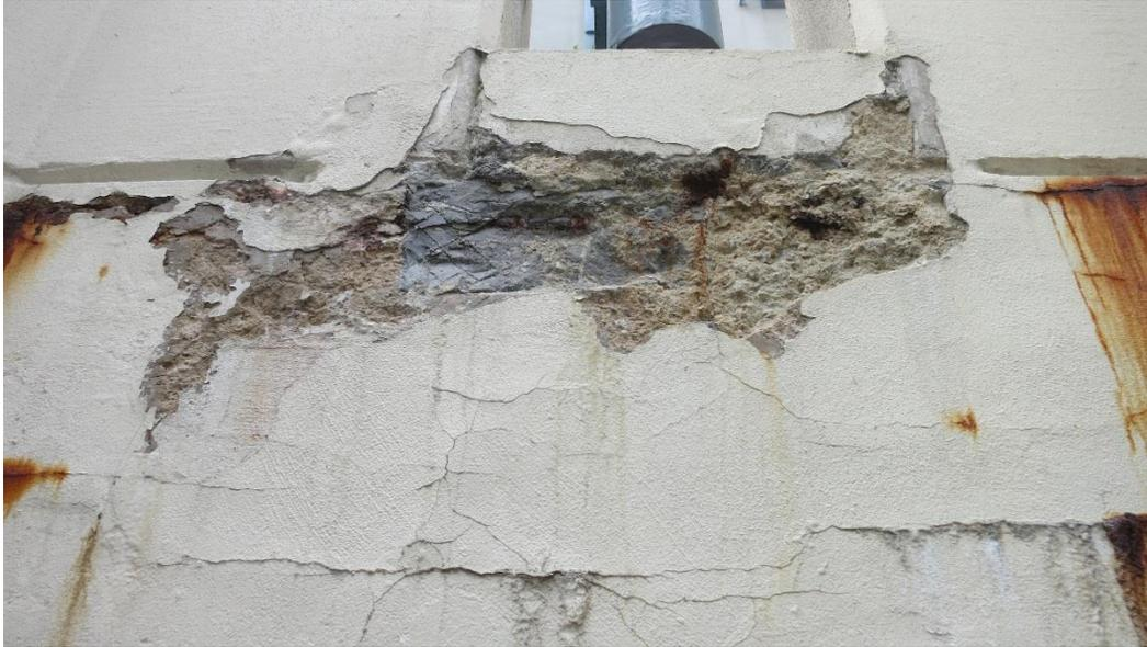
*Photo 7. Spall at lightwell wall*
