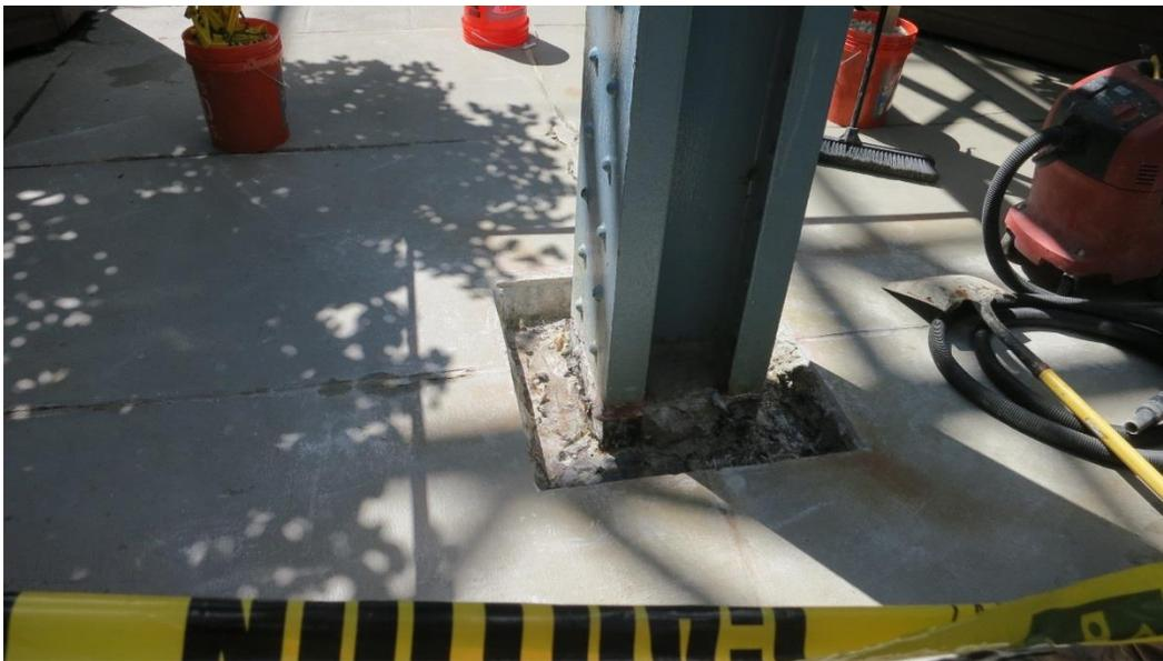
*Photo 16. Probe 7 - Full depth concrete removal at column*
