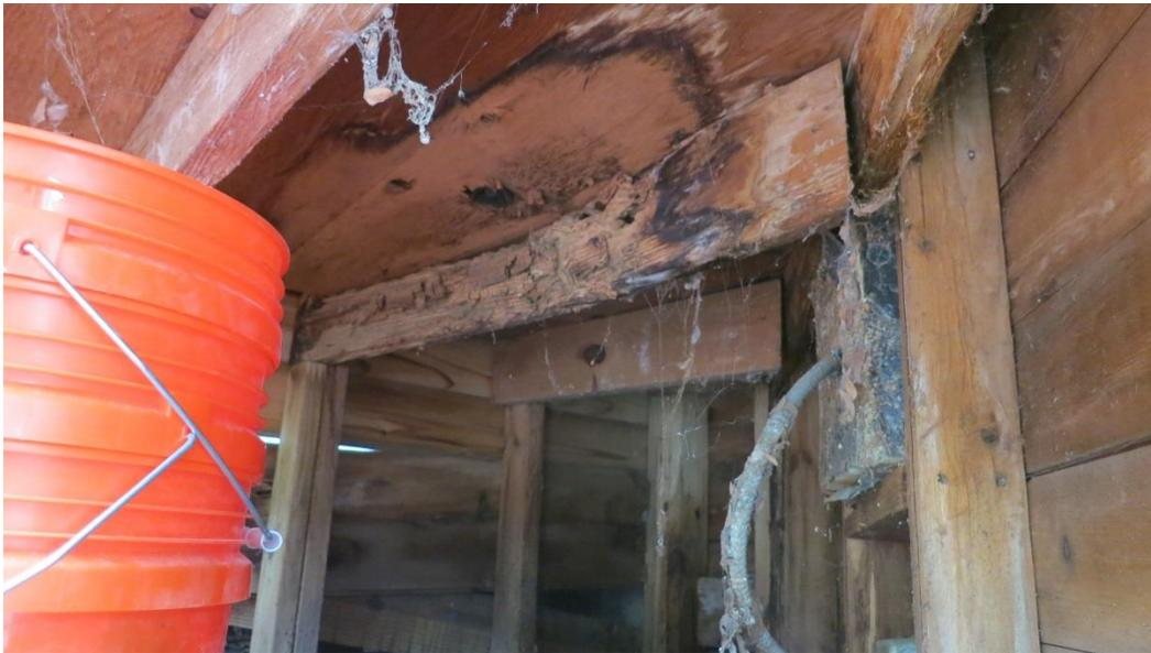
*Photo 26. Deterioration of wood framing beneath planter*
