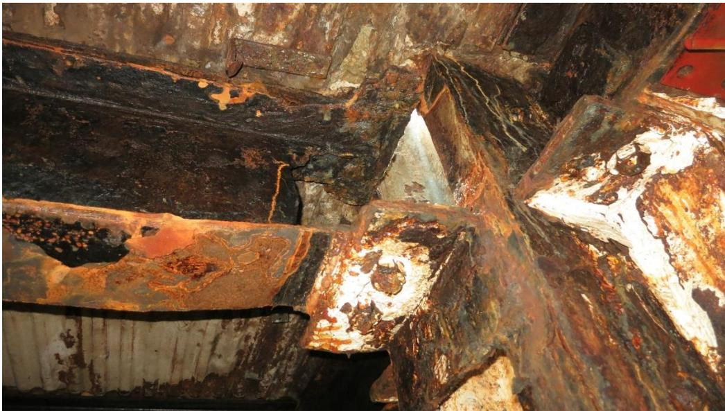
*Photo 2. Corrosion at east column and supported members*
