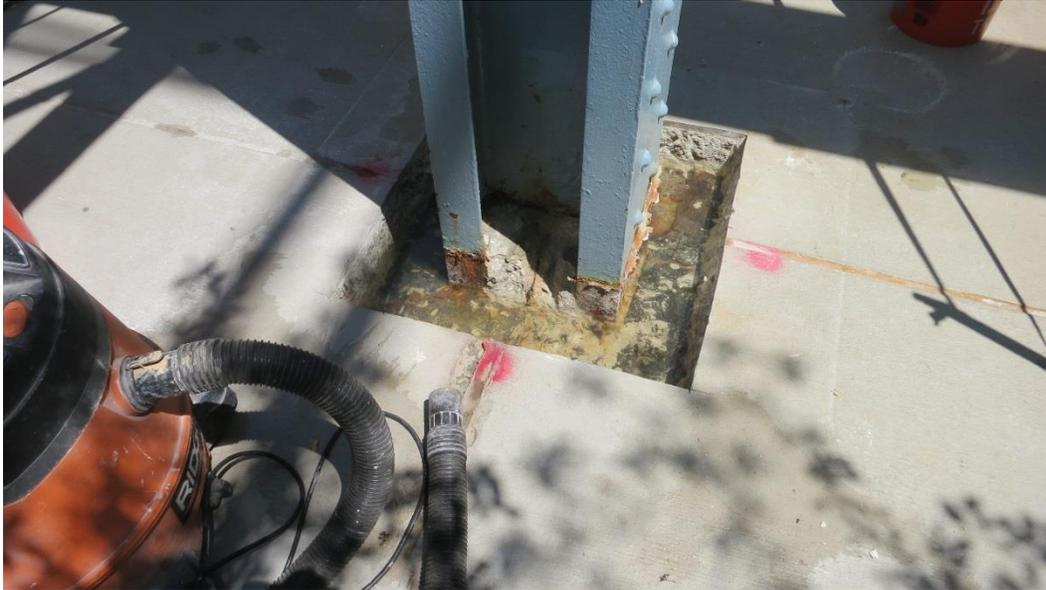
*Photo 15. Probe 6 - Full depth concrete removal at column*
