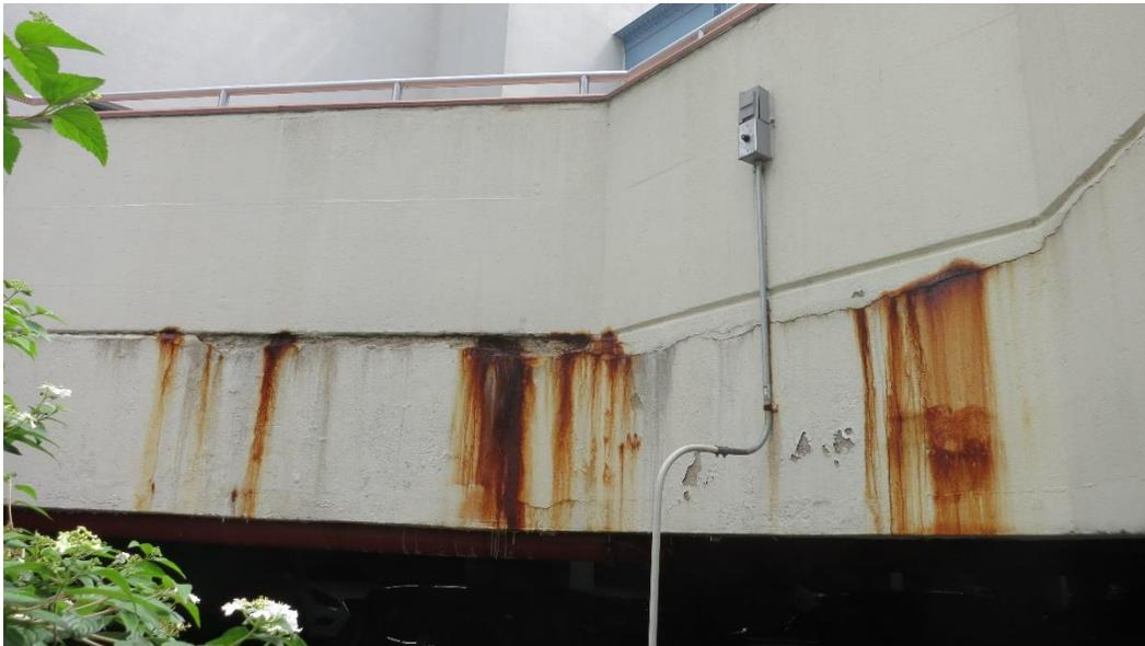
*Photo 6. Stains, cracks, and spalls at lightwell walls*
