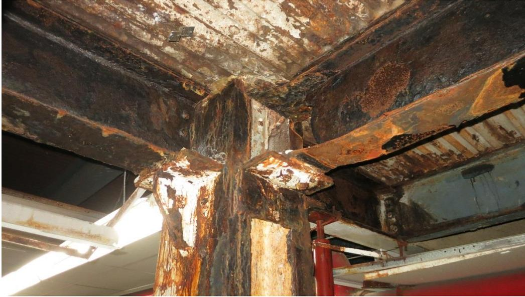
*Photo 1. Corrosion at east column and supported members*
