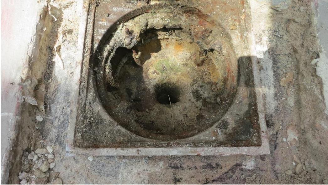
*Photo 17. Probe 8 - Topping slab removal at drain*
