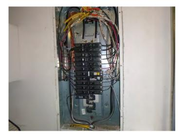
Comments: AFCI (Arc Fault Circuit Interrupter) protected circuits were noted at the bedroom outlets. AFCI's are a relatively new safety feature for residential construction that protects the bedrooms of a home from defective wiring or appliances by shutting off the circuit when a defect is noted. The overall condition of the sub-panels was noted to be good with typical wear noted, although:
