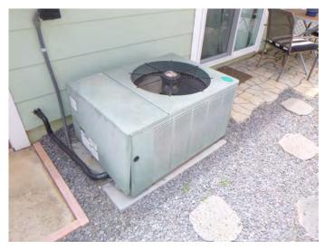
**Comments:** The system was operated and was noted to be functioning properly. The overall condition of the system was noted to be fair with typical wear and corrosion noted, although:
