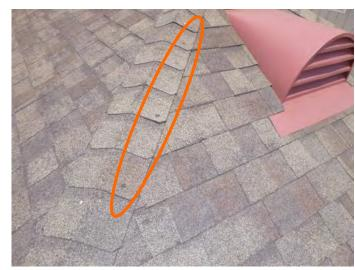
• Several damaged shingles were noted at the back left corner of the roof. This appears to be the result of past vegetation that was in contact with the roof. Contact a licensed roofing contractor for further evaluation and repairs.
