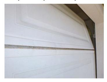
■ Surface corrosion was noted at the exterior of the garage vehicle door. Recommend lightly sanding the affected areas and painting with a rust resistive paint.
