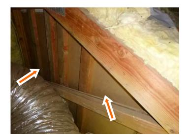
■ Several eave vent screens were noted to be missing or damaged. Recommend installing new screens in order to prevent birds from entering and nesting in the attic.
