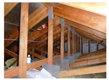
Comments: The hurricane resistance rating for this home could not be determined, as most of the components that affect the rating are not accessible, i.e. most straps, hold down brackets and bracing are covered by exterior and interior wall coverings. Hurricane straps were noted at the trusses in the attic area. This is a component typical for a home of this age. The overall condition of the
