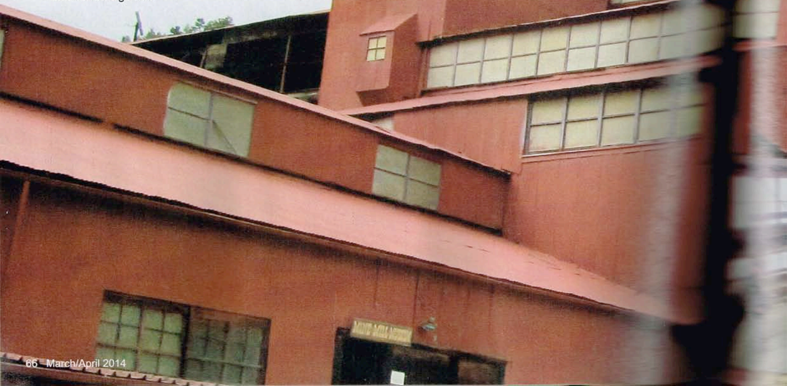
Exterior of Argo Mill.
